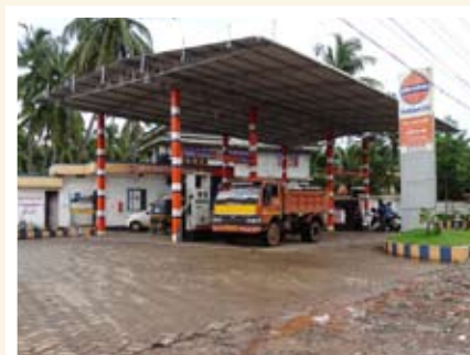
Fuel Station, Padanna
