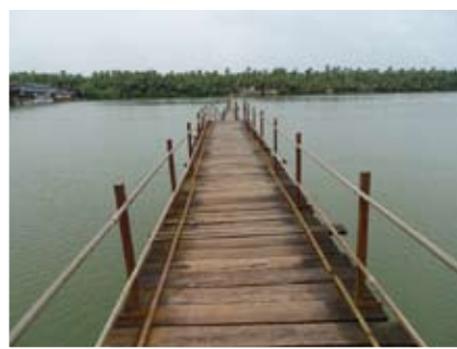
Kottapuram - Achamthuruthi Foot Bridge
