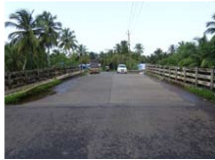
Sultan Canal Bridge
