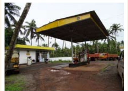
Fuel Station at Thuruthi
