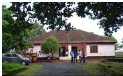
Water Authority guest house, Madayi
