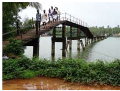
Walking Bridge over Kottapuram
