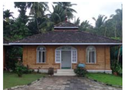
Toilet block at Sargaalaya
