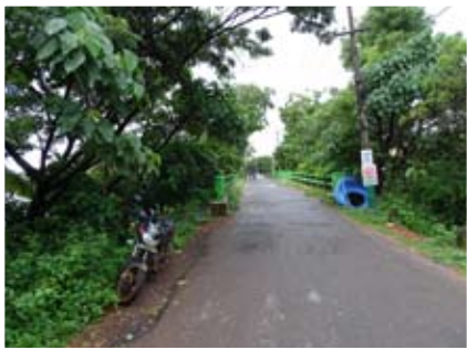
Bridge that connects Kavvayi to the main land
