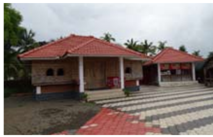
Kadavu Amenity Centre, Edayilekkad
