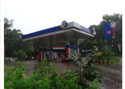
Fuel Station, Edayar
