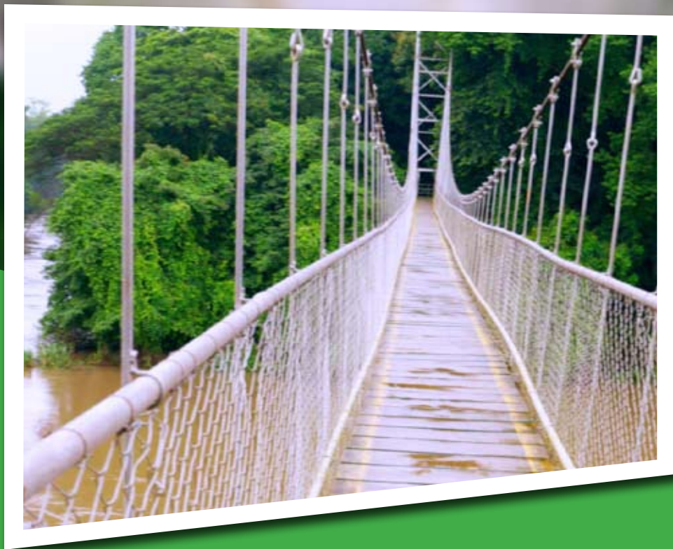
The hanging bridge at Nilambur
