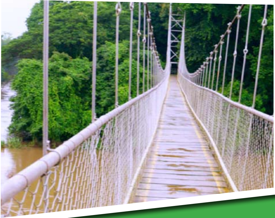
The hanging bridge at Nilambur
