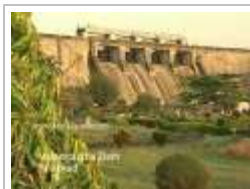
Malampuzha dam in Palakkad
