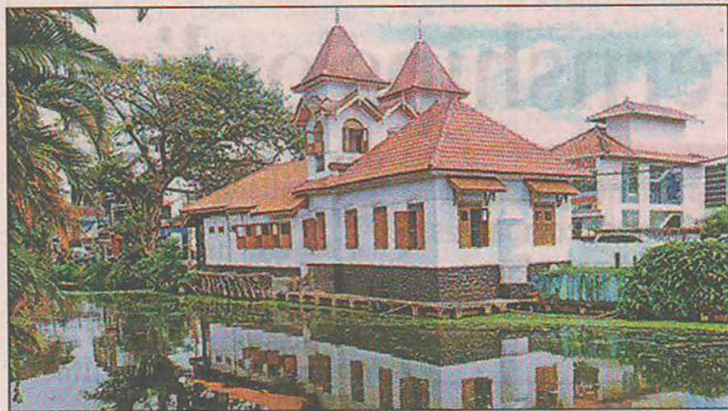
The museum, the first of its kind in the country, is being developed as part of the Alappuzha heritage tourism project. (Above) A heritage building under renovation as part of the project
